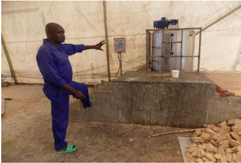
A Soap factory employee explaining how the boiler works
