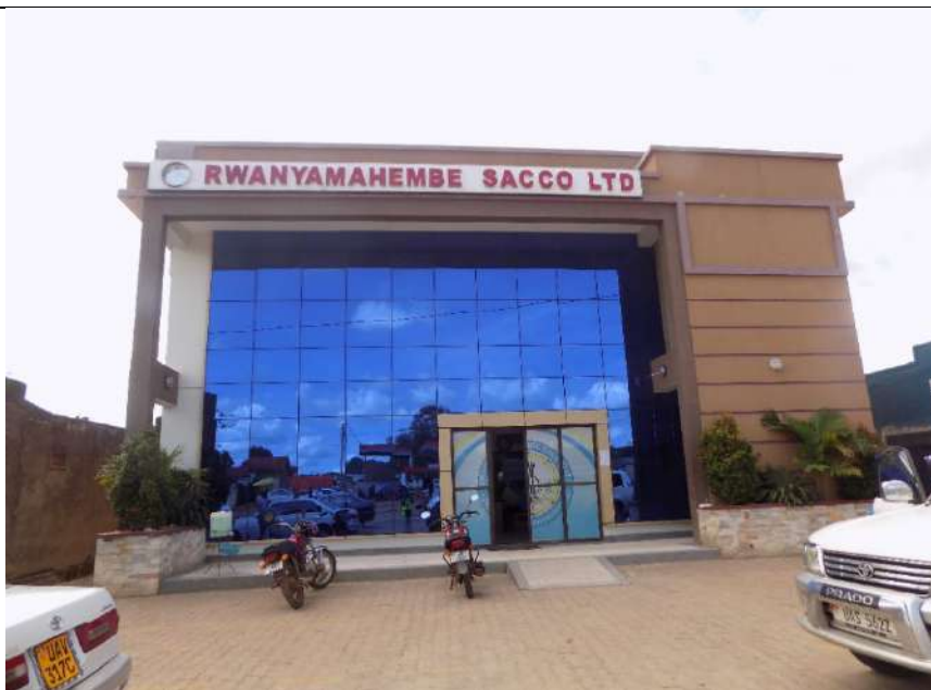
Head office in Buzibwera town along Ibanda- Mbarara road
