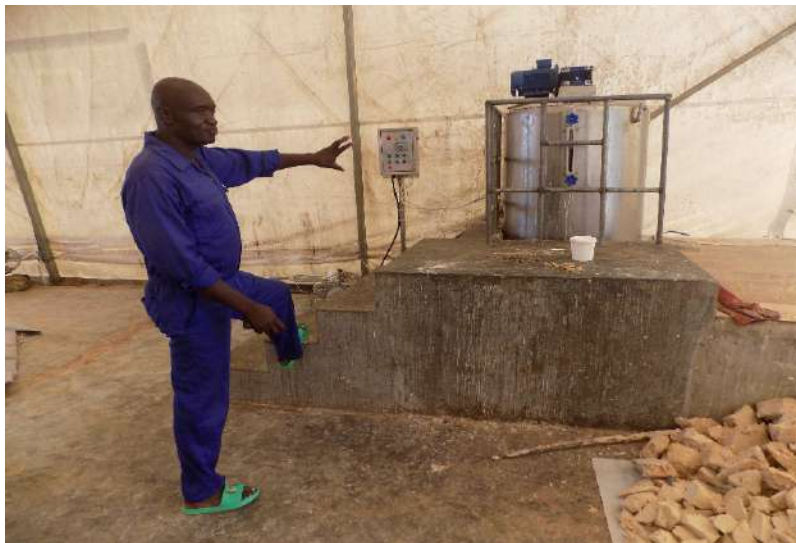
Figure 0-7: Soap factory employee explaining how the boiler works, (Photo by JBN, Nov. 2022)
